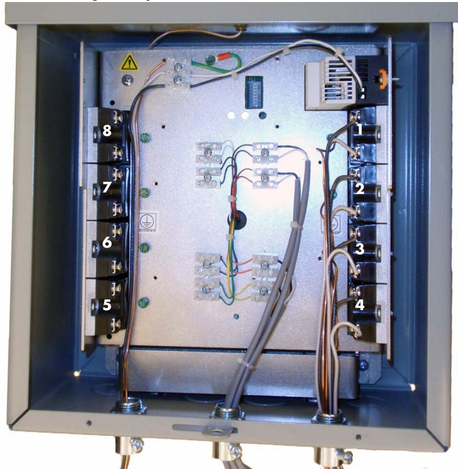
FIGURE 6. Numbering of relay terminals
